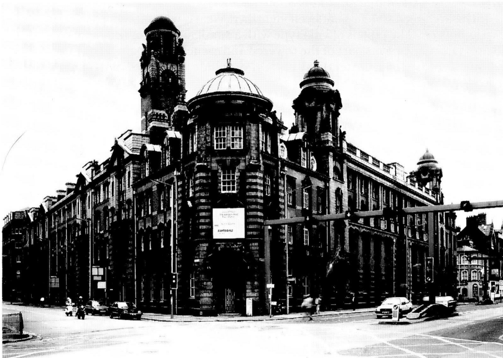
Fig. 7 Central Fire Station, Manchester RCHME Crown Copyright
